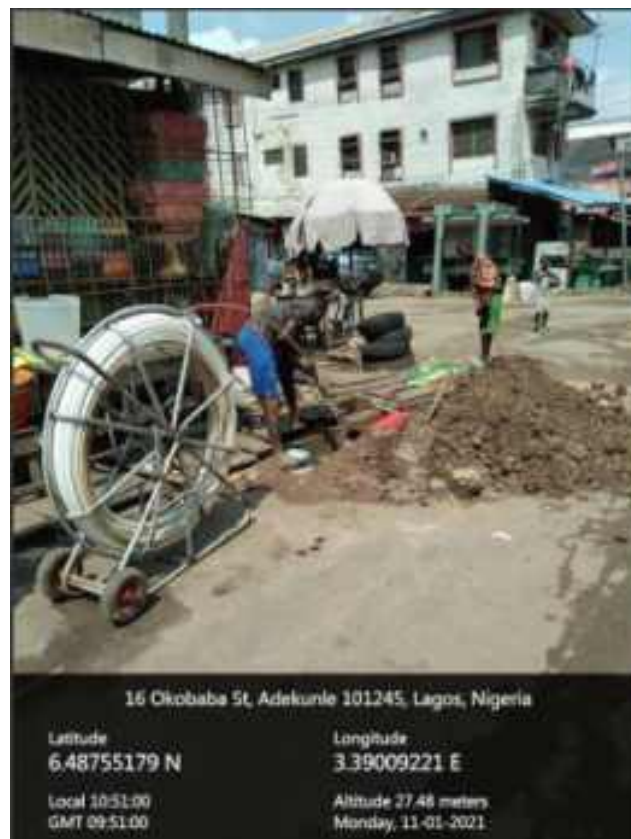
Duct rodding for fiber pulling
