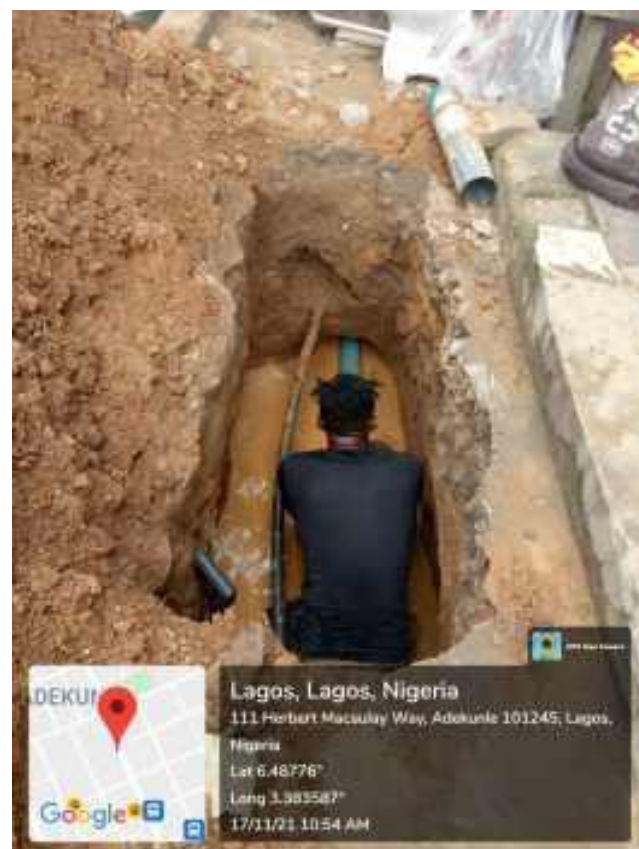
Thrust boring manual method
