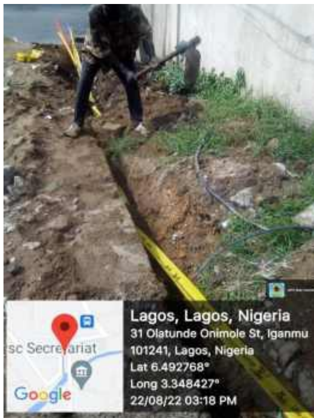
Open trenching backfilling for METRO
